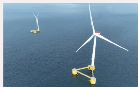
Figure 1 Example of a semi-submersible floating substructure. Photo of the WindFloat Atlantic project courtesy of Principle Power/Ocean Winds.
