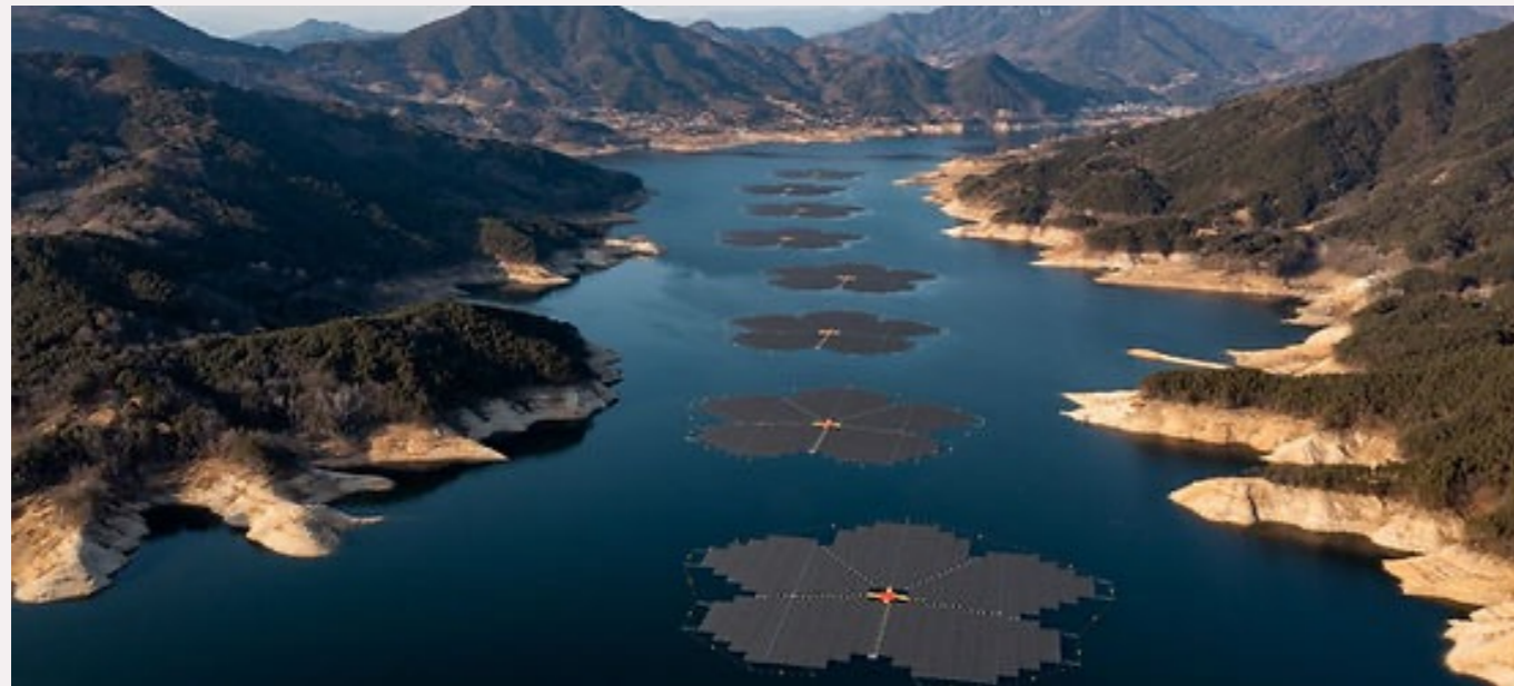
Figure 1: Floating solar panels on the surface of the Hapcheon Dam in South Korea. The project can generate enough to power 20,000 homes, according to Hanwha Solutions. Source: Bloomberg Photographer: SeongJoon Cho/Bloomberg
